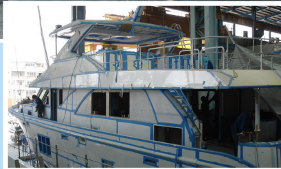
New Build Inspection
