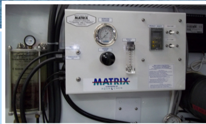
Installation of Matrix 1400gpd Watermaker
