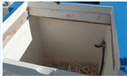
Fiberglass Demolition to allow for Larger Gas Grill
